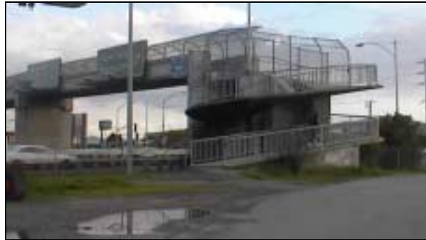
Nellen Avenue Overcrossing
