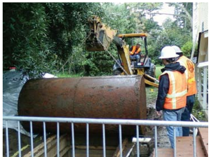
Inset: A County employee receives hazardous materials training. Above: An underground fuel tank is carefully removed.
