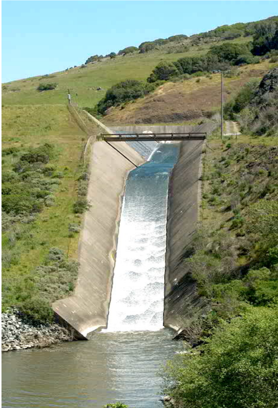
Lake Nicasio Spillway April 18, 2005
