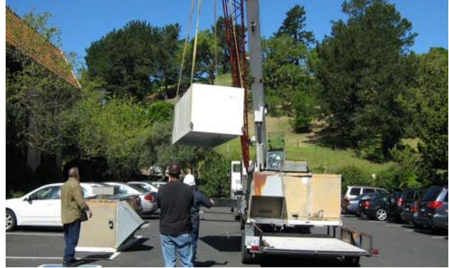
10 North San Pedro HVAC replacement
