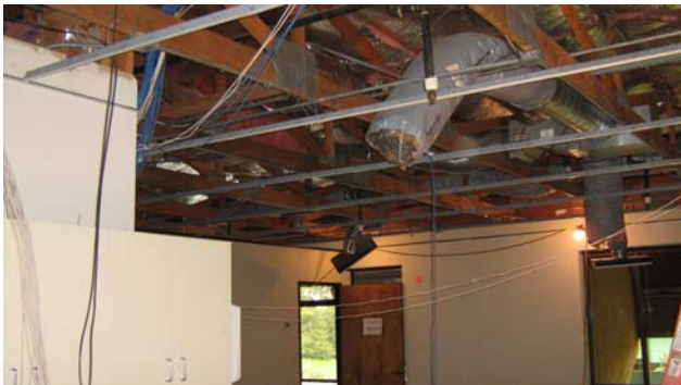
10 North San Pedro interior demolition
